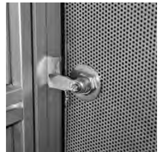
panel firmly bolted together
